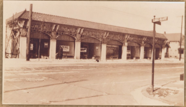
Oakland Avenue and Lake Bluff Boulevard construction, ca. 1922.
