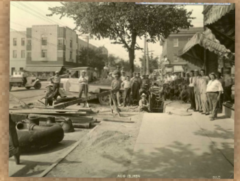
WPA street crew, Oakland Avenue and Capitol Drive, Aug. 13, 1934.
