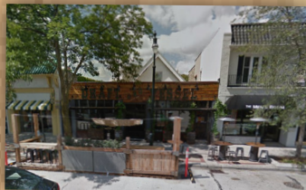
2017 – Draft & Vessel occupies entire storefront and includes a street parklet for additional seating.
