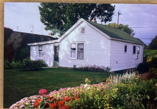
The original two-room farm house located at 4525 N. Oakland Ave. was built about 1870. Despite efforts to save it, it was razed in 2004.
