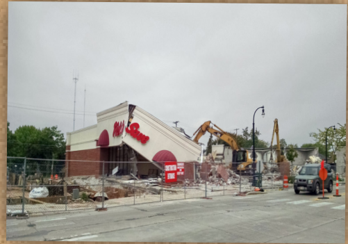
Demolition of Pick 'n Save on Oakland Avenue in Shorewood, 2016.
