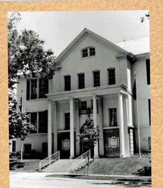
The first major renovation of Village Hall was completed by WPA workers in the late 1930s. Along with an addition to the back of the building, columns and other decorative elements were added to give the building a colonial look which was popular at the time.
