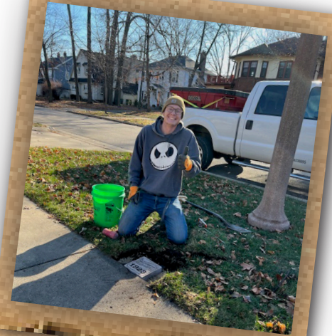
Adam Nichols from Envision Outdoor Services installs a new Birthday Marker on the 2100 block of E. Olive Street. Birthday Marker installations were a bit behind schedule but better weather on Dec. 7, 2023 helped move things along. (Photo credit: Clancy Carroll)
