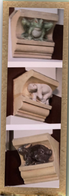
Above: New corbels of critters were reproduced by Continental for the 1929-30 addition to Lake Bluff school to match the originals from the 1924 section of the building.
