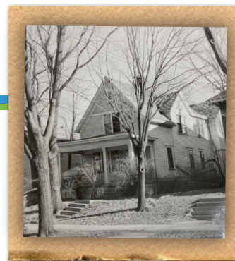
House at 4146 N. Murray Ave. prior to remodeling in 1960.
