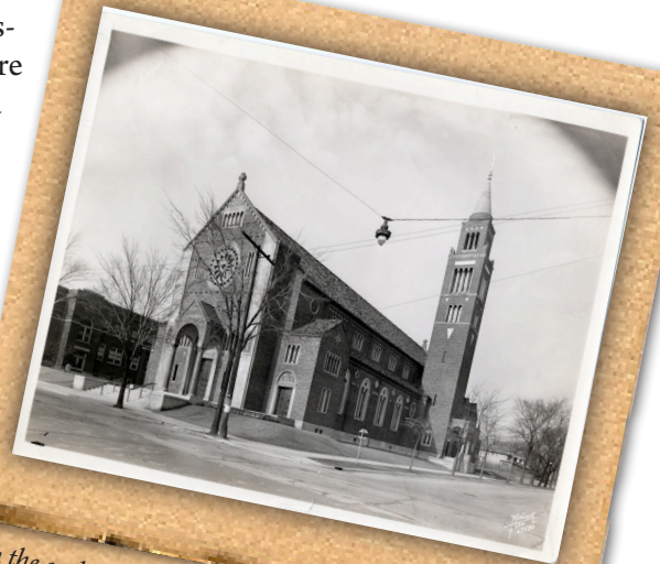
In the early 1940s the intersection street lights were hanging on wires suspended over the area. This light was near St. Robert's Church at the intersection of Capitol Dr. and Farwell Ave. Note the electric utility poles near the curb.
