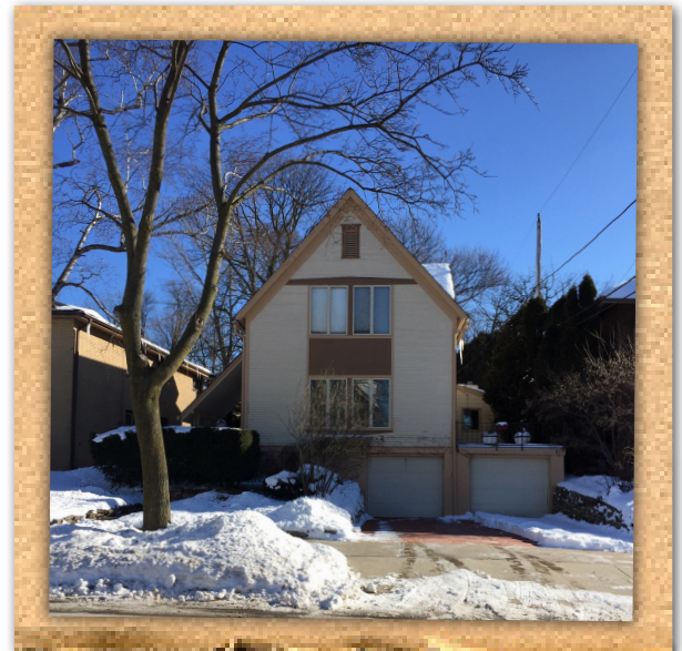
Present day picture of the renovated home at 4146 N. Murray Ave.
