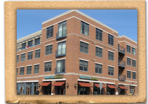
The Cornerstone Apartments at 4507 N. Oakland Ave. is also home to Colectivo Coffee and other retail.
