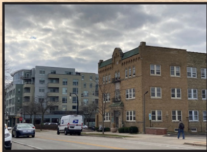
An example of two stages of apartment development along Oakland Ave. near the Olive St. intersection. The Mosaic is in the background and the Stratford Apartments, 4221 N. Oakland Ave., is in the foreground.
