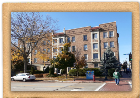
3953 N. Maryland Ave. is an example of the apartments that were built along Capitol Dr. in the mid-1920s to early 1930s.
